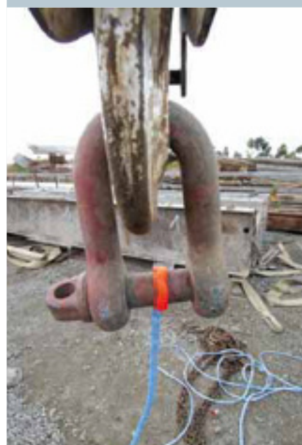
The crane driver takes up the slack
